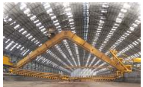
Portal Scraper Reclaimer
