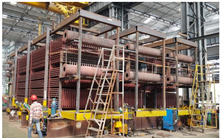
PH Boiler Coil Module Under Fabrication
