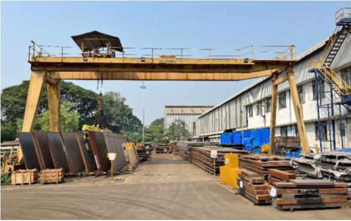
Yard – Efficient Storage
